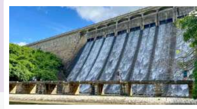
大潭上水塘水壩 Tai Tam Upper Reservoir Dam
