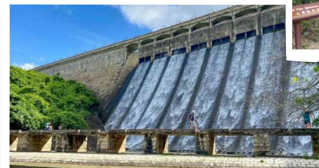
大潭上水塘水壩 Tai Tam Upper Reservoir Dam
